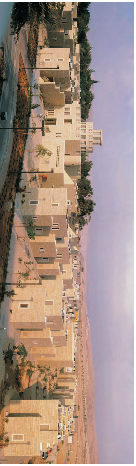
▼ The outdoor spaces were designed to receive direct sunlight from south according to the “Sun Envelope” for the short winter days. The topography is slanted inwards to collect run off water and to divert it towards the vegetation. Deciduous trees were chosen to achieve maximum shade in the summer and to allow for the sun to penetrate in the winter.
